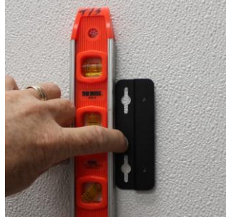
Figure 3 - Marking Holes for Vertical Mounting Bracket
